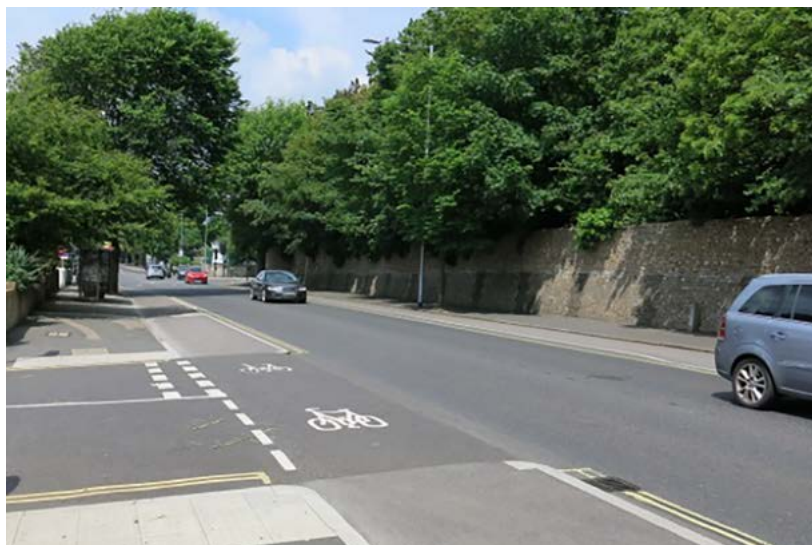
Stepped cycle track at side road junction
